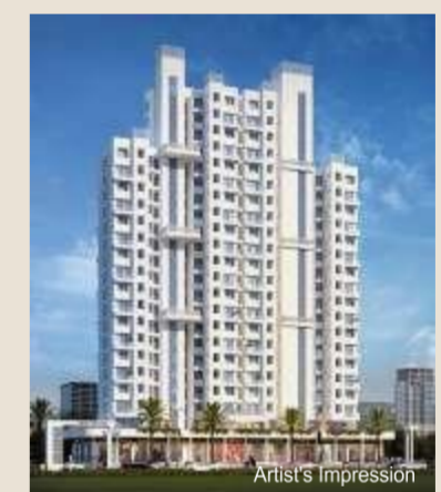
ONGOING PARTH SKYONE DOMBIVLI - EAST
