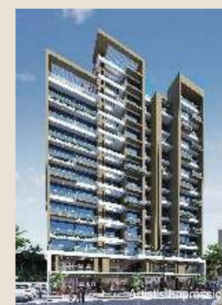
COMPLETED PARTH MAGNUS SANPADA, NAVI MUMBAI
