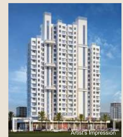
ONGOING PARTH SKYONE DOMBIVLI - EAST
